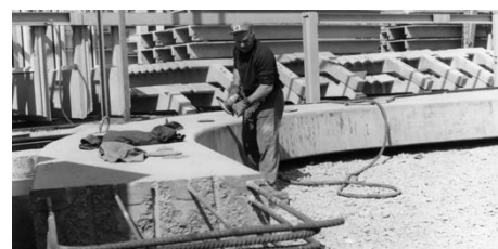
Figure 9 Concrete Arches during construction (Photo by: Alvar Aalto Foundation) Seeing photographs of the process of the construction is always important. Observing the progress of a man working on the beam is quite impressive, seeing the methods used. and satisfying. This photo offers a clear view of the interior of a reinforced concrete beam and its curved design.
